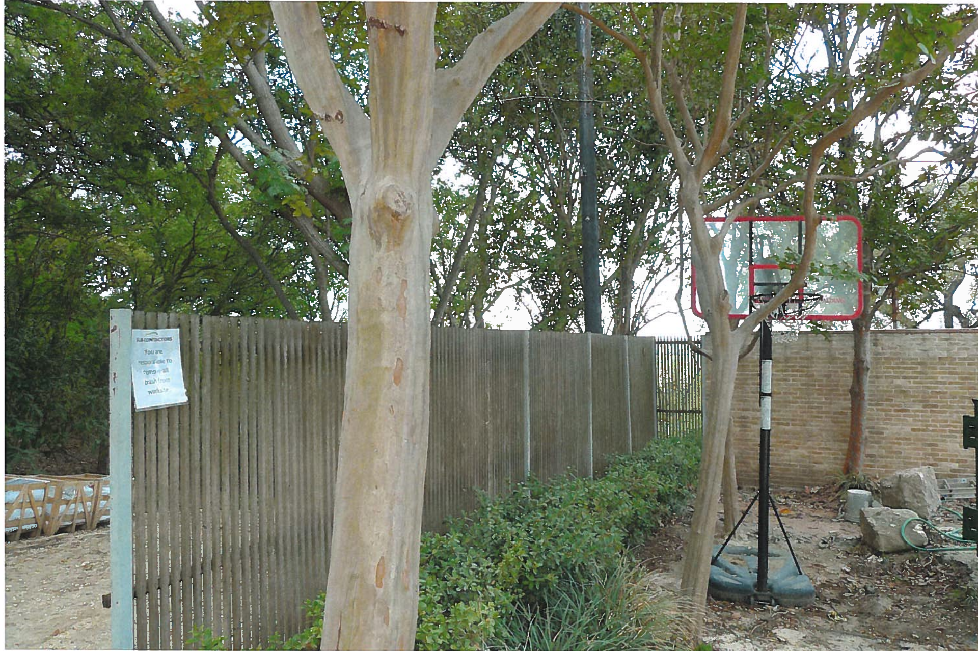
EXISTING FENCE (ALIGNS WITH BOTTOM OF WALL CAP OF EXISTING BRICK WALL)
